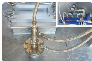
라임분사노즐 Lime Injection Nozzle
